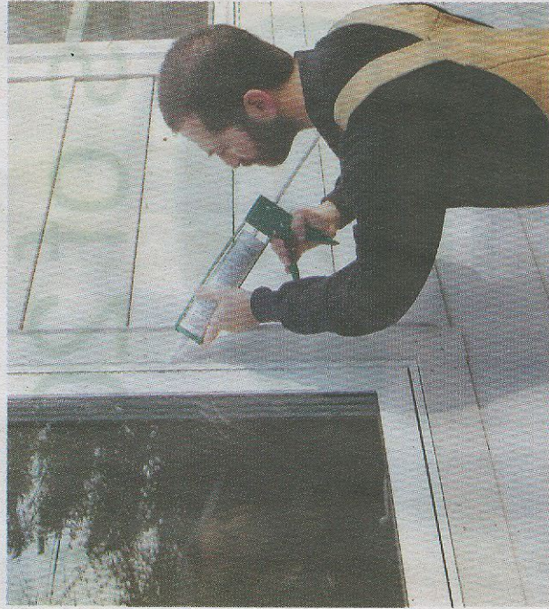
Ron Flax, project manager of Skycastle Homes, a remodeling contractor that "greenmodels" homes affordably, installs caulking to a window frame to prevent air infiltration. Air leaks can account for between 25 to 40 percent of the heating and cooling cost of a home.
